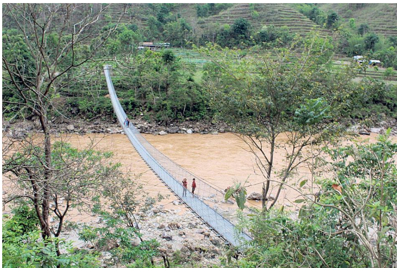
Trail Bridge near Benighat and Siddhalek Villages, Dhading, Source: Republica, 2018
